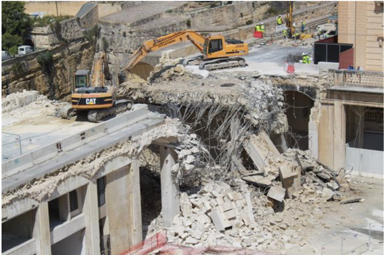
Valletta gate demolition, photo Riet Eeckhout.
